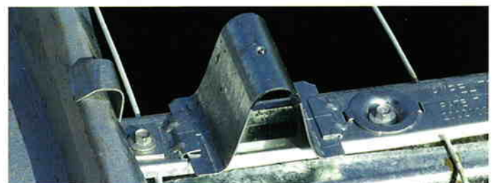
ClearSlide decking support ready to be crimped to deck.
