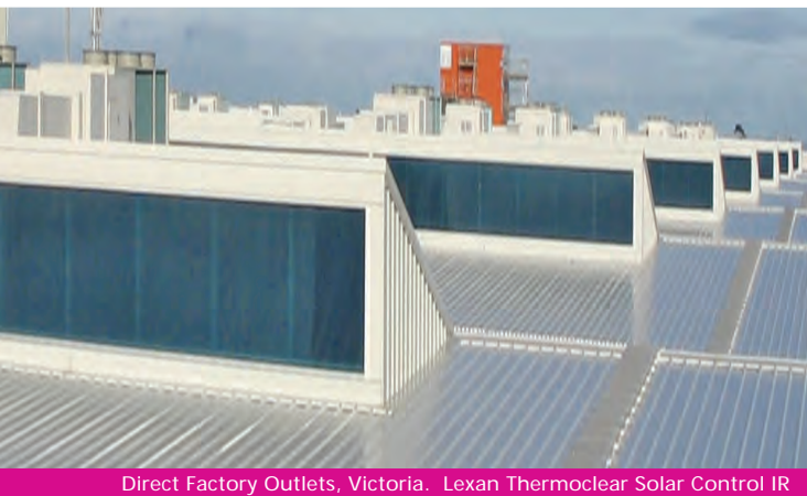
Direct Factory Outlets, Victoria. Lexan Thermoclear Solar Control IR
