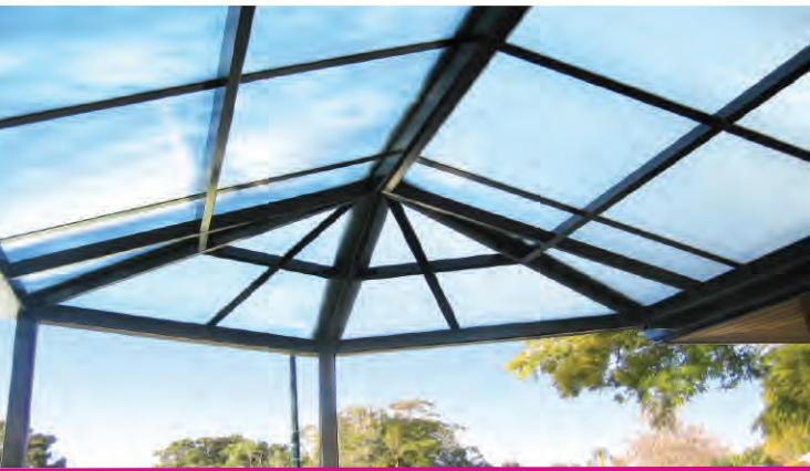
Residential pergola, Victoria. Lexan Thermoclear 10 mm opal
