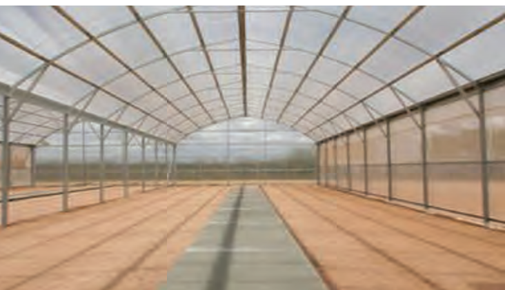
Quarantine Greenhouse, Victoria. Lexan 8 mm Clear Photo courtesy Redpath Ideal Greenhouses
